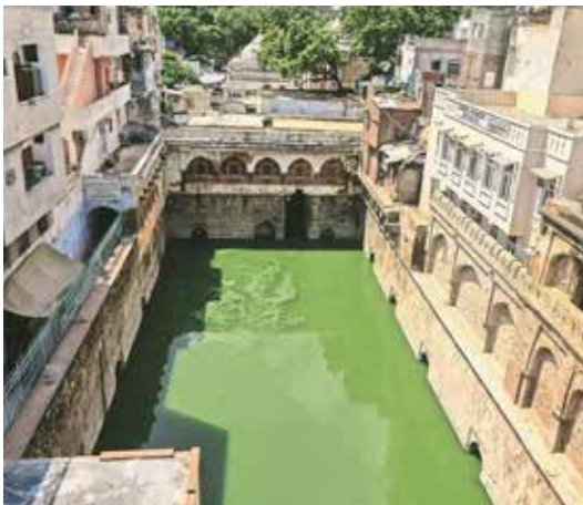
AKDN Nizamuddin Basti - Delhi, India: Renewal Project
